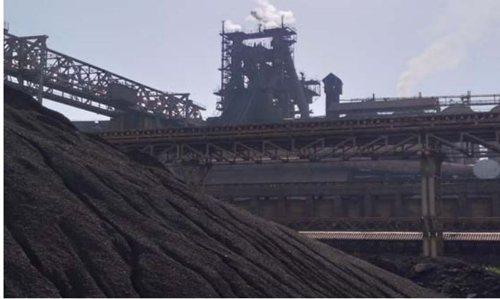
Figure 4. Eastern layout view from a broken portal crane
