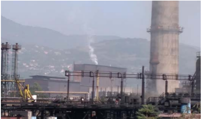
Figure 3. Western layout view from a broken portal crane
