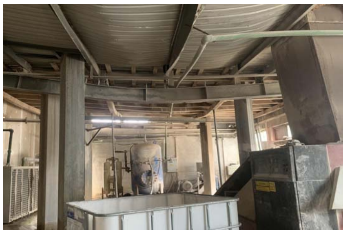
Figure 12. Detailed position of plastically deformed sections & roof
