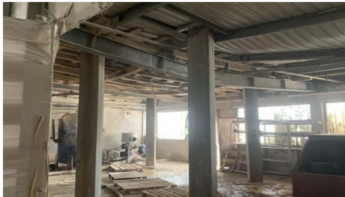
Figure 11. Position of the wooden section supports to plastically deformed sections & roof
